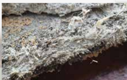
THE TROUBLE WITH ASBESTOS
